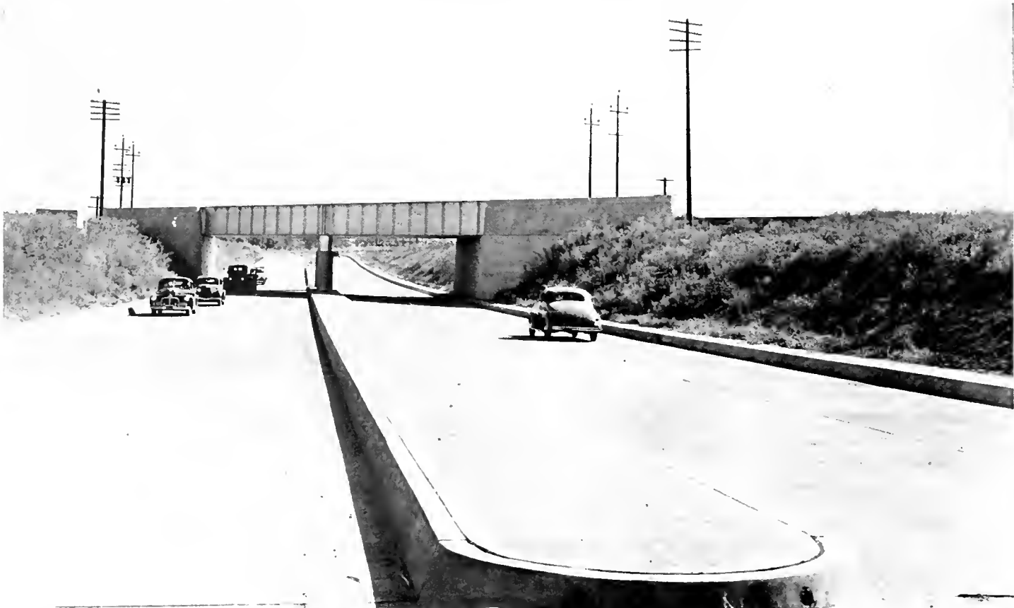
Four-lane divided underpass on Davis-Dixon cut-off where the Southern Pacific Railroad crosses the highway. This structure is one of the modern features which permit a saving of 150,000 vehicle hours annually
